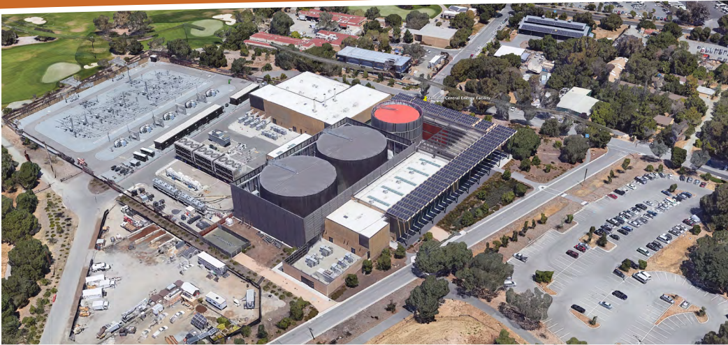
Stanford University's decarbonization strategy includes three large water tanks for thermal energy storage at their Central Energy Facility. | Google Earth. Maps Data: © 2021 Google.
