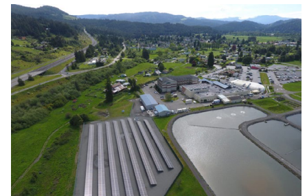
Blue Lake Rancheria Microgrid (Schatz Center, Cal Poly Humboldt)
